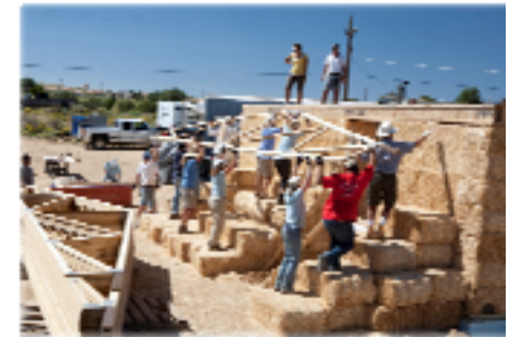
Volunteers work together to raise the tresses for the roof.
